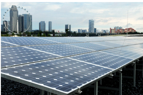
Picture courtesy of PUB The largest Solar Park in Singapore at the Marina Barrage covers an area of 1,200sq m. The 405 solar panels generate electricity used for indoor lighting and power points in the Marina Barrage.
