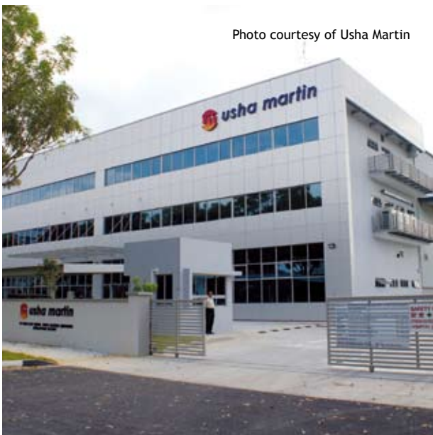
The Usha Martin regional headquarters in Singapore. The company has grown from strength to strength, to become a global conglomerate with major global presence
