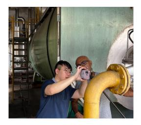
Setting up multiple phones on tripods as a low-cost method to validate key metrics of steam production and consumption. This informs the level of instrumentation required for the product.
