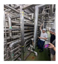
Testing the feasibility of low-cost Infrared imaging cameras to identify causes of water hammering problems within heat exchangers, at a beverage processing plant in Singapore.
